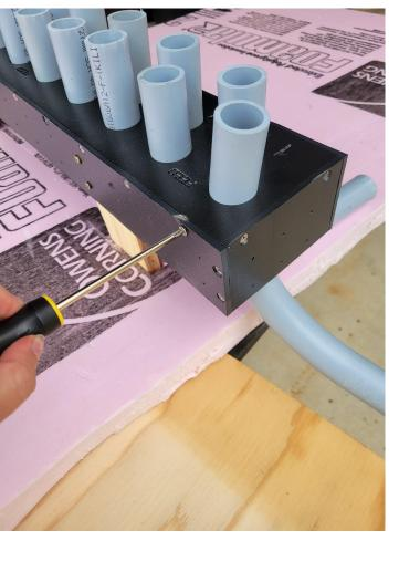
3. The H4 elbows come in the standard front position, all elbows facing out and as high as the elbows can go. Each elbow has a screw that locks it into place.
