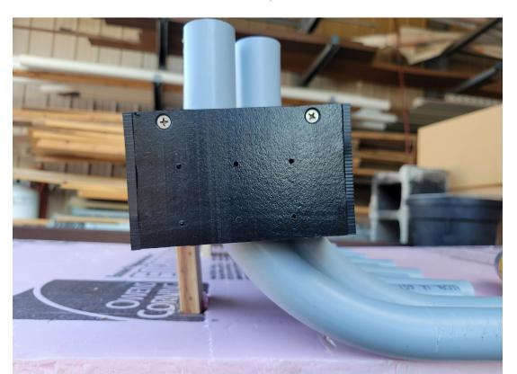
6. Run your pex pipes, according to the plan you have made, beginning and ending each 300' run by running it through the matching elbow on the H4.
