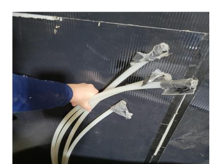
Put tape on the hose ends to prevent debris from entering them while you are building and before they are hooked up to the HUG Hydronics unit.
