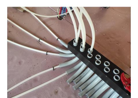
In this picture you can see the little black staples holding the pex tubes in place. They are typically used every 1-4 feet to keep pex in place while pouring cement.
