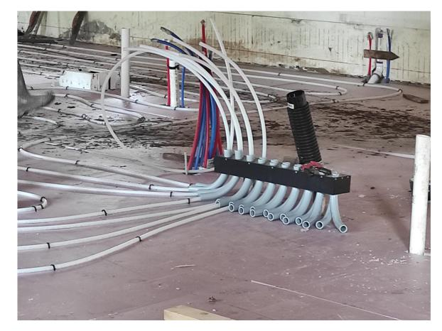
7. When all the Pex pipes are laid you may want to tape the tops of the hoses to prevent debris from falling into them.
