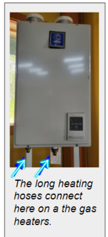
Graphic 17) Gas Water Heater Hose Connection
