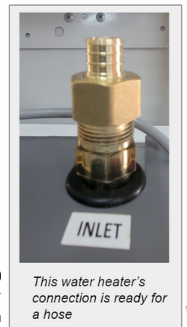
Graphic 6) Water Heater Connection
