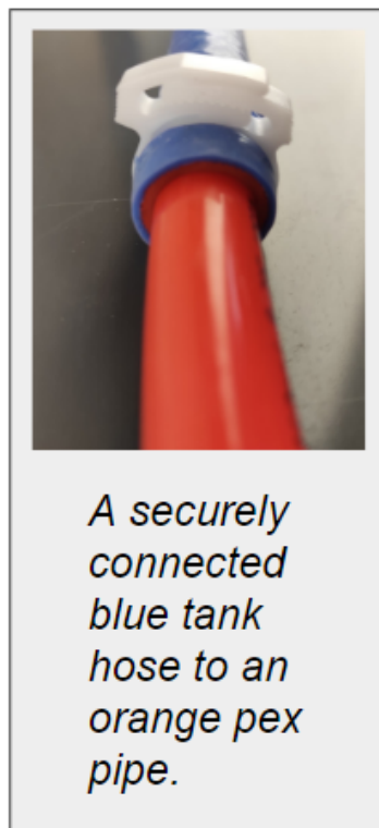
Graphic 13) Completed Hose Connection
